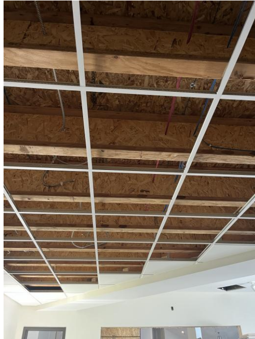
Photo #2: Ceiling Grid Install in the Lobby
