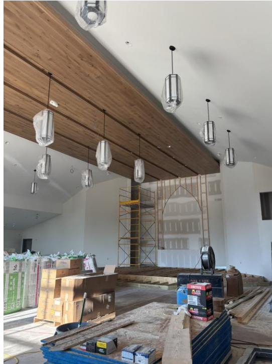
Photo #3: Alter Platform Rough Framing
