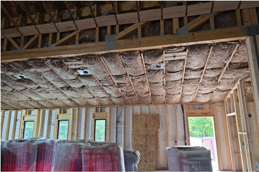
Photo #2: Insulation Install
