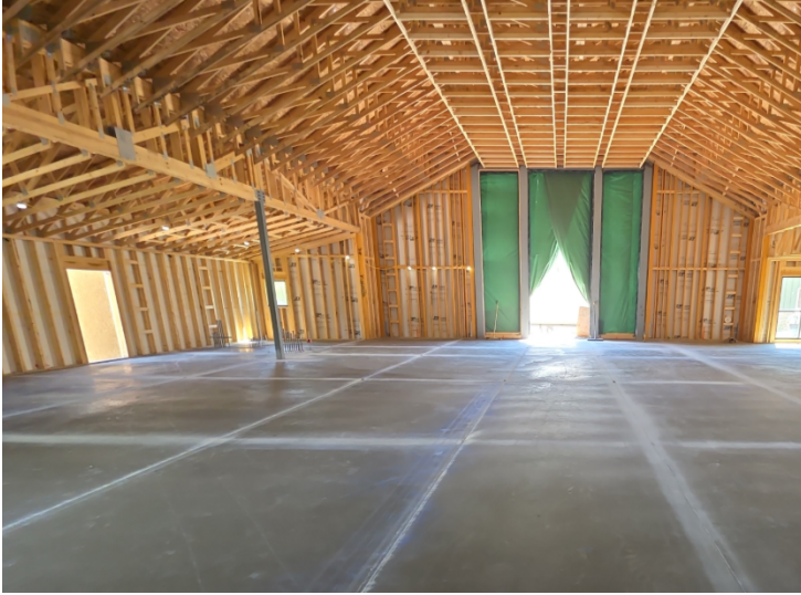
Photo #2: Slab joints
